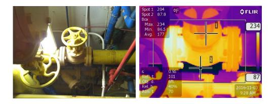
Low Pressure Steam Valve Operating Temperature, \*F Ambient Temperature, \*F Insulation selected
